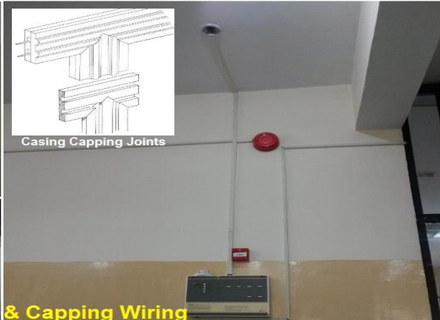
Casing & Capping Wiring
