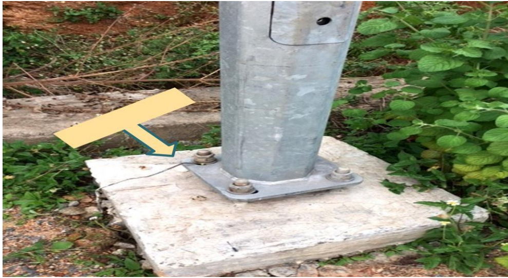
Fig.2.23. Strip Earthing
