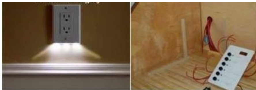
Fig.2.9. Concealed conduit wiring.
